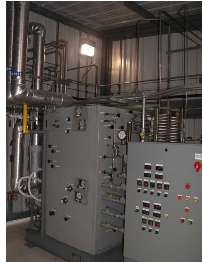
Picture of an MPT membrane test skid at NCCC for testing hydrogen separation by carbon molecular sieve membrane modules with shifted syngas.
